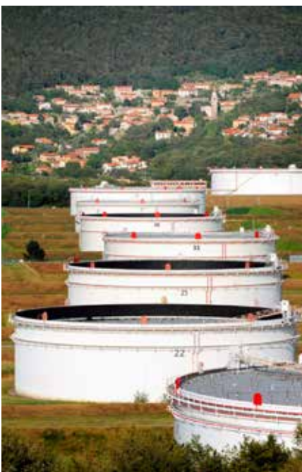
Transalpine Pipeline – Tanklager Triest.
